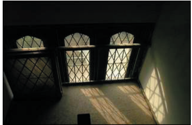
The Charles P. Moorman Home for Women will keep its original windows as it's converted into the Inverness Condominiums.
